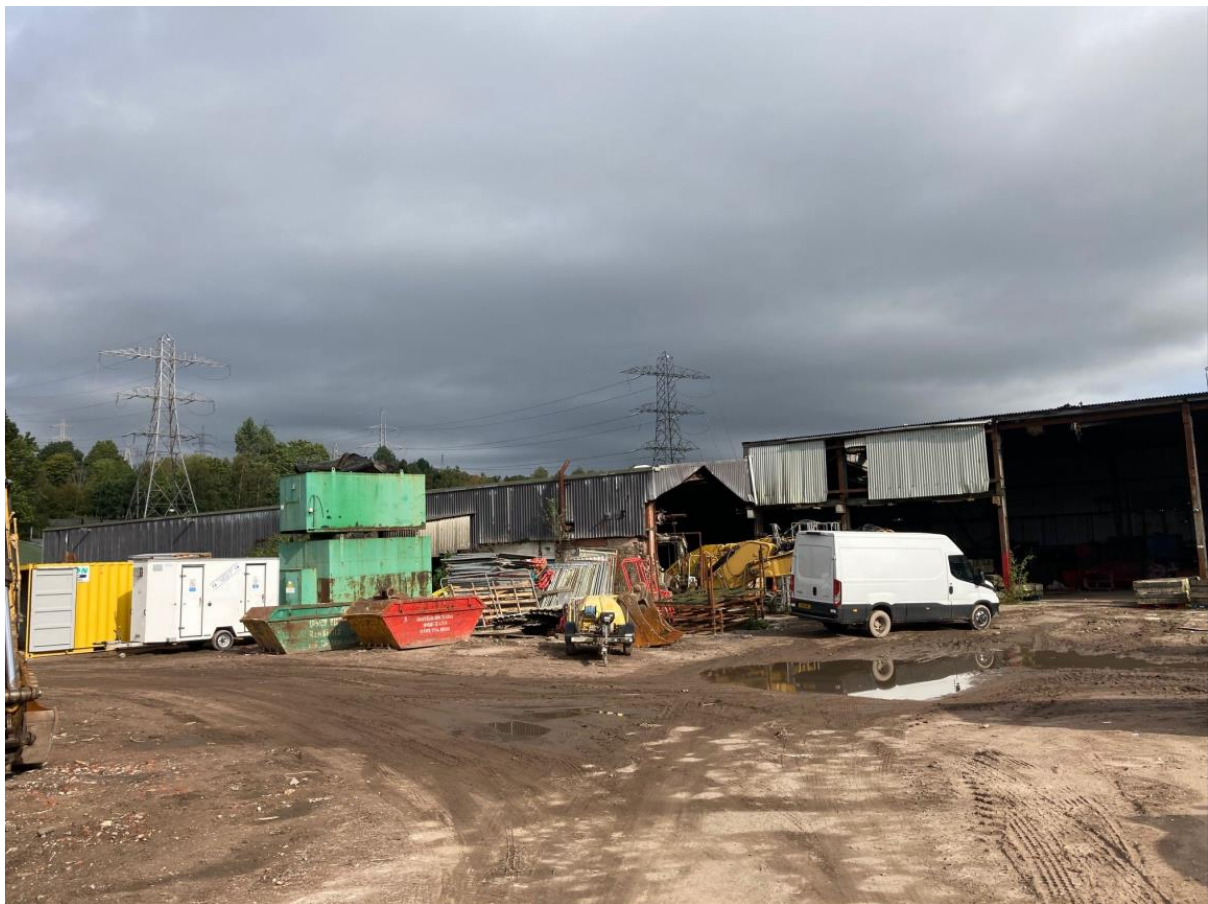
Photo 5: View across site from Northend Road bridge
