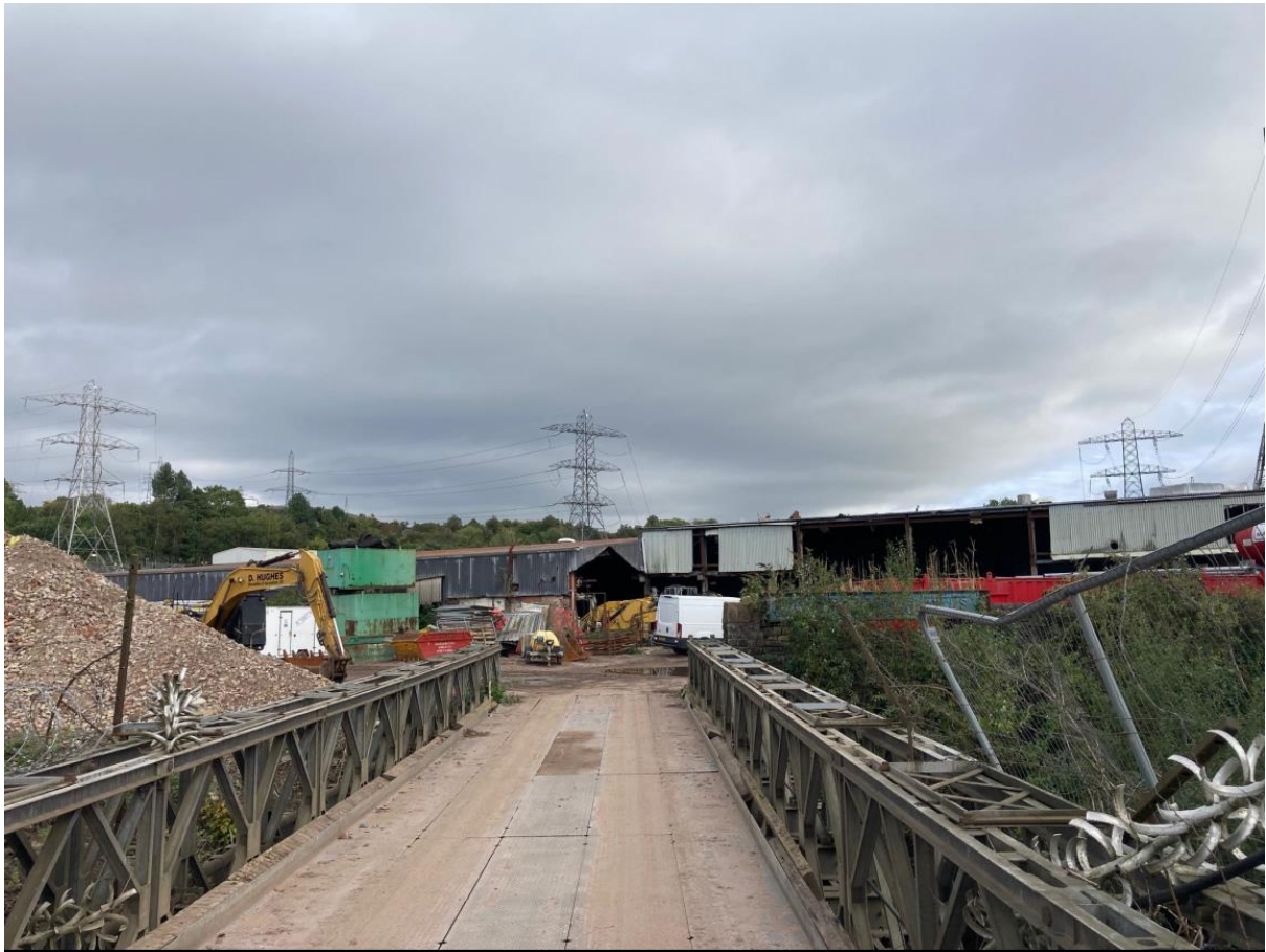
Photo 4: View towards site from Northend Road
